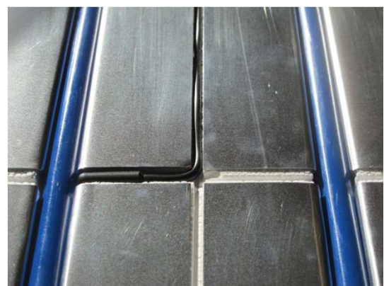
JUPITER IDEAL element showing positioning of floor sensor
